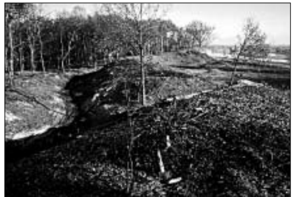
Figure 4. Removal of wildshoots to improve the visibility of this 11 th century fortress wall
